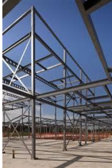
The steel “skeleton”
